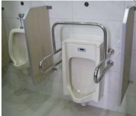
Urinal designed for the disabled (automatic flush sensor)
