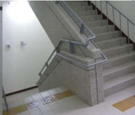
Accessible staircases for the blind in every building (blind guidance and handlebars)
