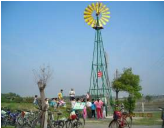
Water pumping windmill
